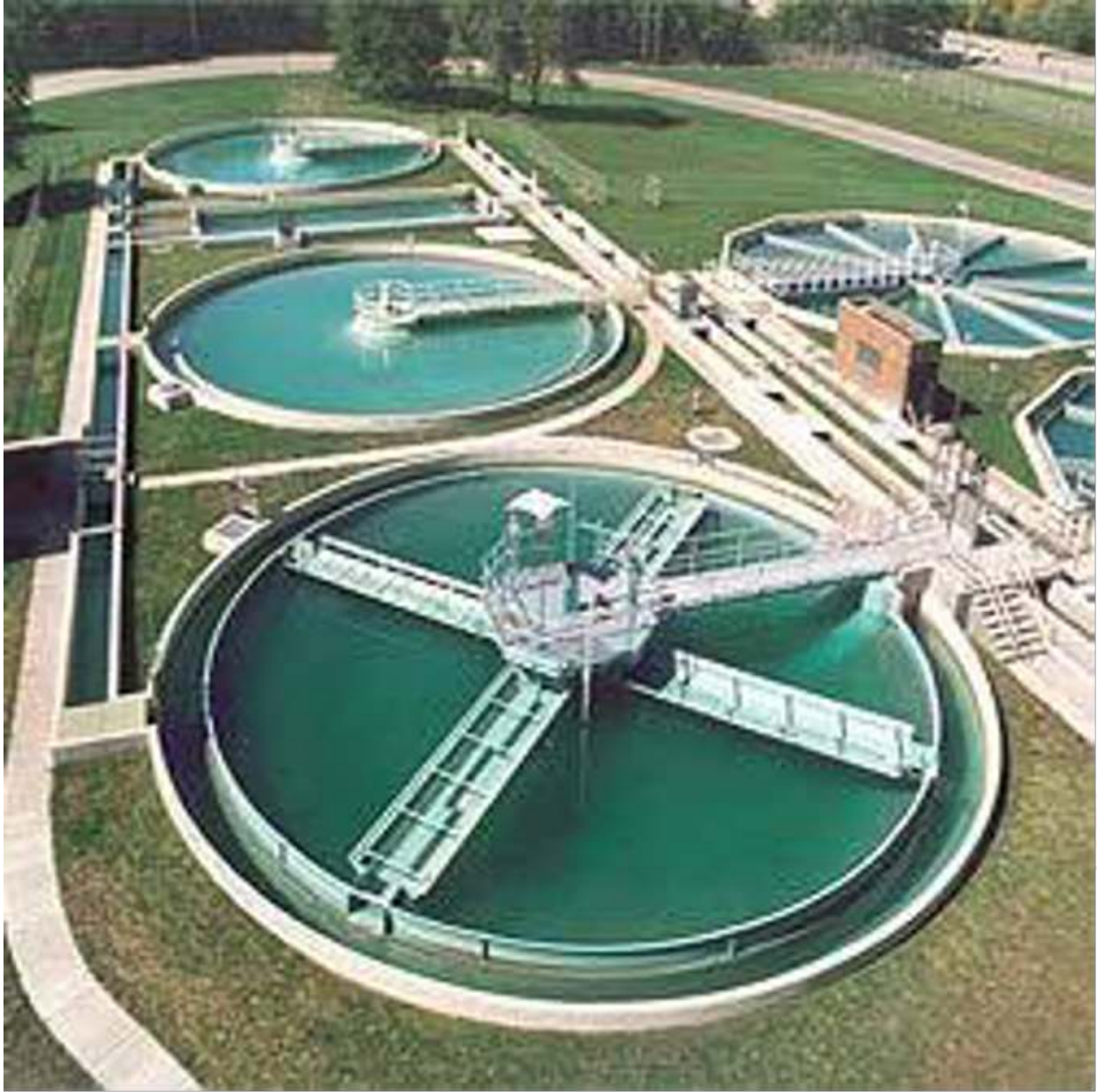
E.L. SMITH Potable Water Treatment Plant CLARIFIER TANKS
