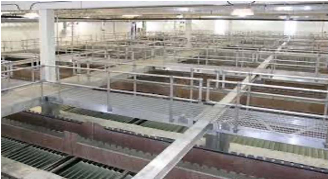
GOLD BAR WASTEWATER TREATMENT PLANT – CLARIFIER TROUGHS
