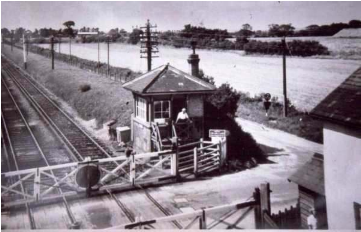
YAPTON CROSSING SIGNAL BOX (FRED OSBORNE STANDING AT THE DOOR) FRIDAY 10 FEB 2017
