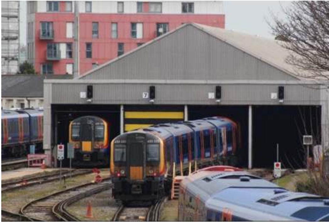
FRATTON TRAIN CARE DEPOT, PORTSMOUTH, HAMPSHIRE
