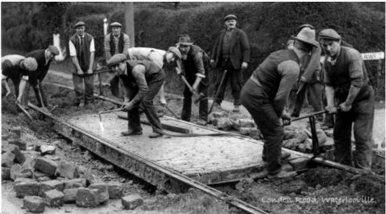
Removal of the tramway tracks, London Road, Waterlooville, 1935.
