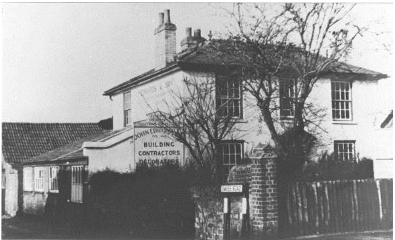
Bury (Berry cottage) Cottage. First described as Bury Cottage in a sales particular for May 1840 when it was described as a 'neat and modern and well manufactured house'. It was demolished to make way for the new Post Office.
