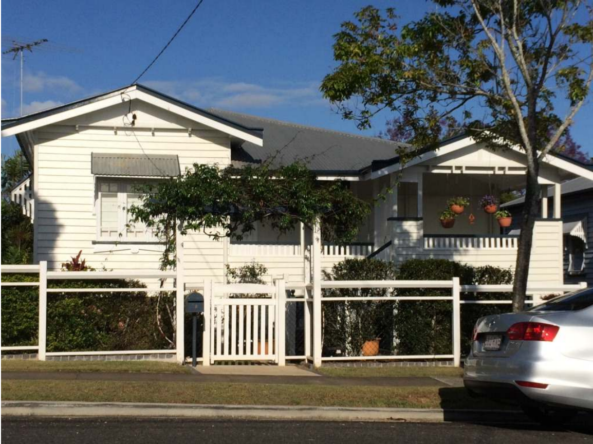
ERNEST MONK'S House in Ashgrove, Brisbane, Queensland, Australia.
