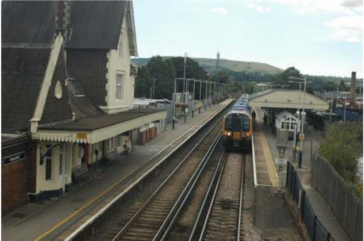
PETERSFIELD STATION, Hampshire
