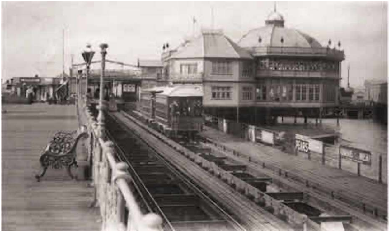
RYDE PIER STATION – Electric Train
