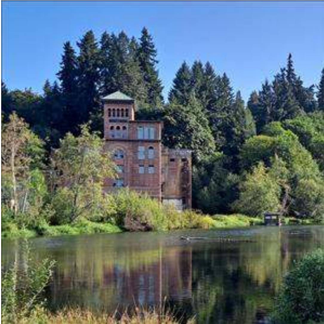
Old Brewhouse (Olympia Brewing Company, 1906), Deschutes River, Tumwater. Photo by Colleen E. O'Connor, ca. 1860 Courtesy Washington State Historical Society
