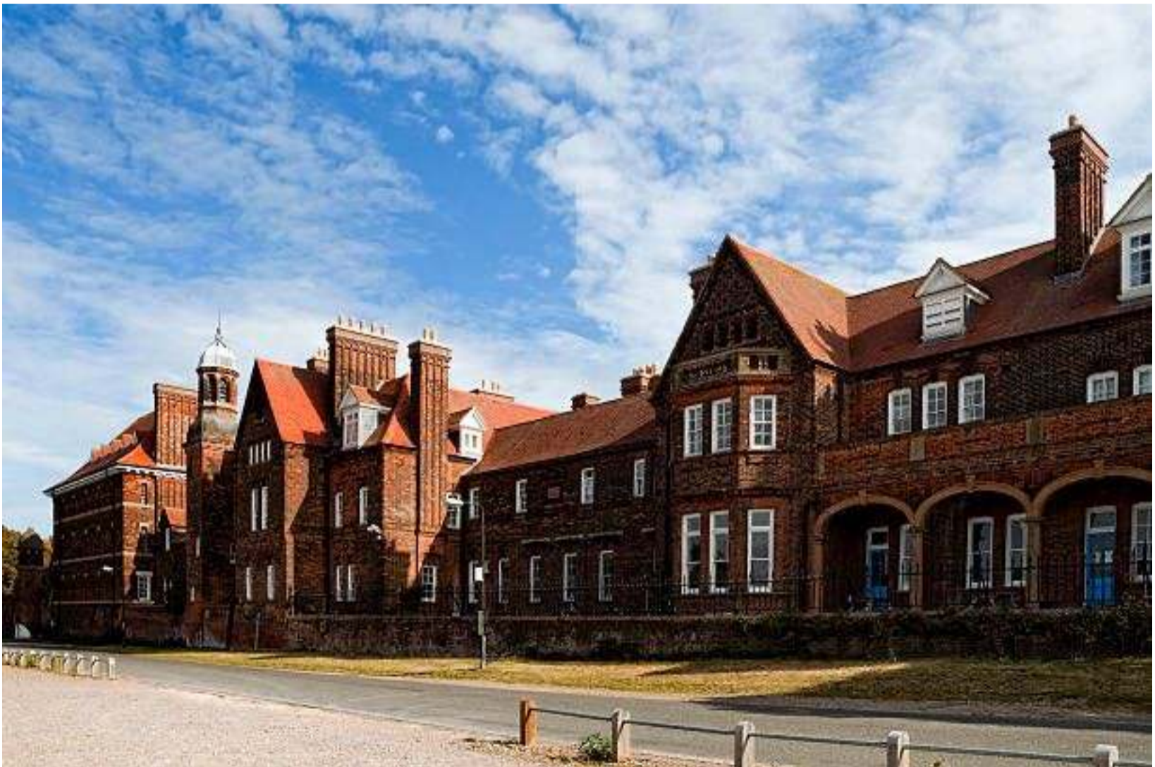
Britannia Barracks, Norwich.
